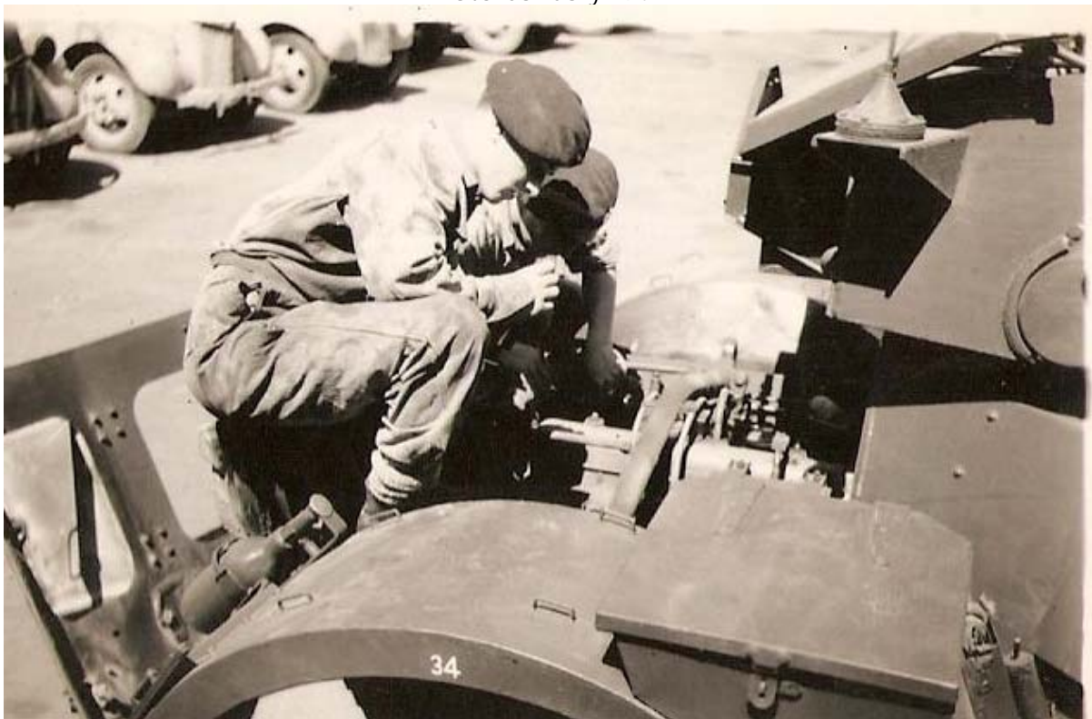
Photo Courtesy of Photographer : Lance Corporal John (Jack) Clifford Location: Egypt, Abyssia, Cairo Description: Daimler armoured car F339461 named CAVALIER, Crewman George Lane & Smudger Smith of 1trp, check the plugs. Date: March 1947
